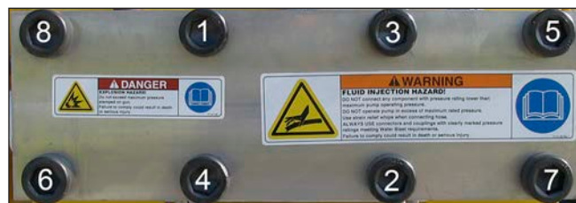
Figure 44: Tightening Sequence.
