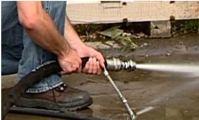
Fig. 27: Flushing the Discharge Hose
