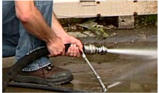
Fig. 6: Flushing the Discharge Hose
