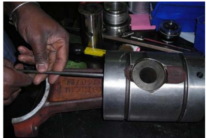
Figure 170: Second Set Screw Installation.
