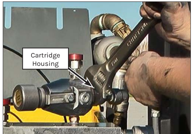
Figure 131: Cartridge Housing Removal.
