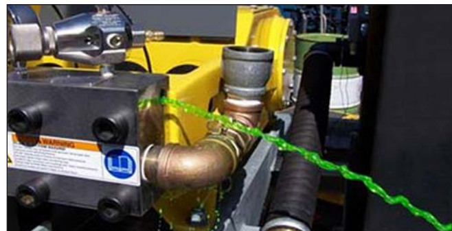
Figure 44: Draining the Anti-Freeze.
