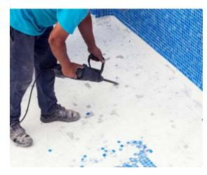
The conventional method of sandblasting, chipping, or jackhammering to remove old pool plaster is an application of the past. These traditional methods of replastering are expensive, ineffective, and cause severe damage to the pool shell.
